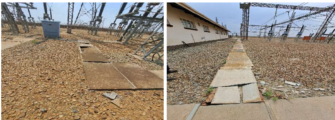
Current condition of the trench covers
